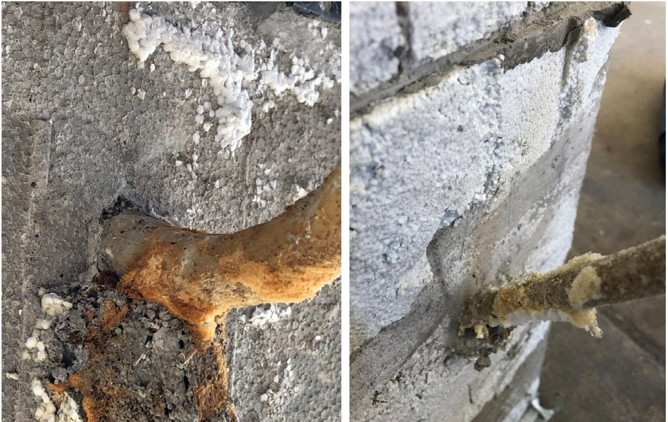
*Figure 9 Spar attachments to concrete wythes*
